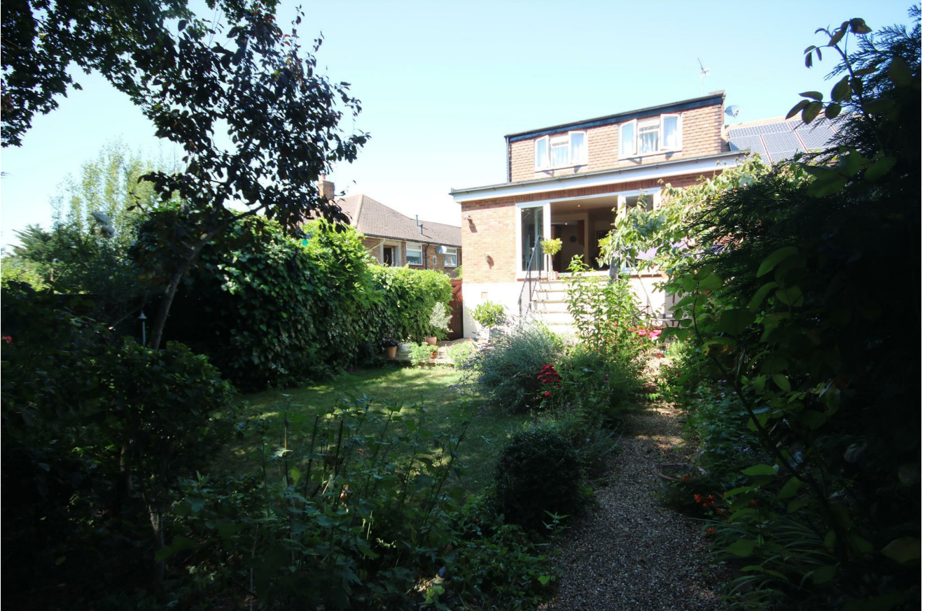
REAR ELEVATION OF PROPERTY:
